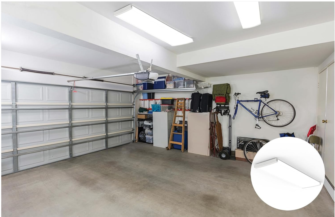
Image 10.1: TruWrap fixture providing illumination in a garage.
