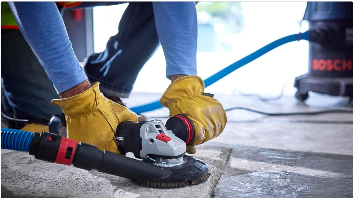
Figure 4: Angle grinder in use for concrete grinding.
