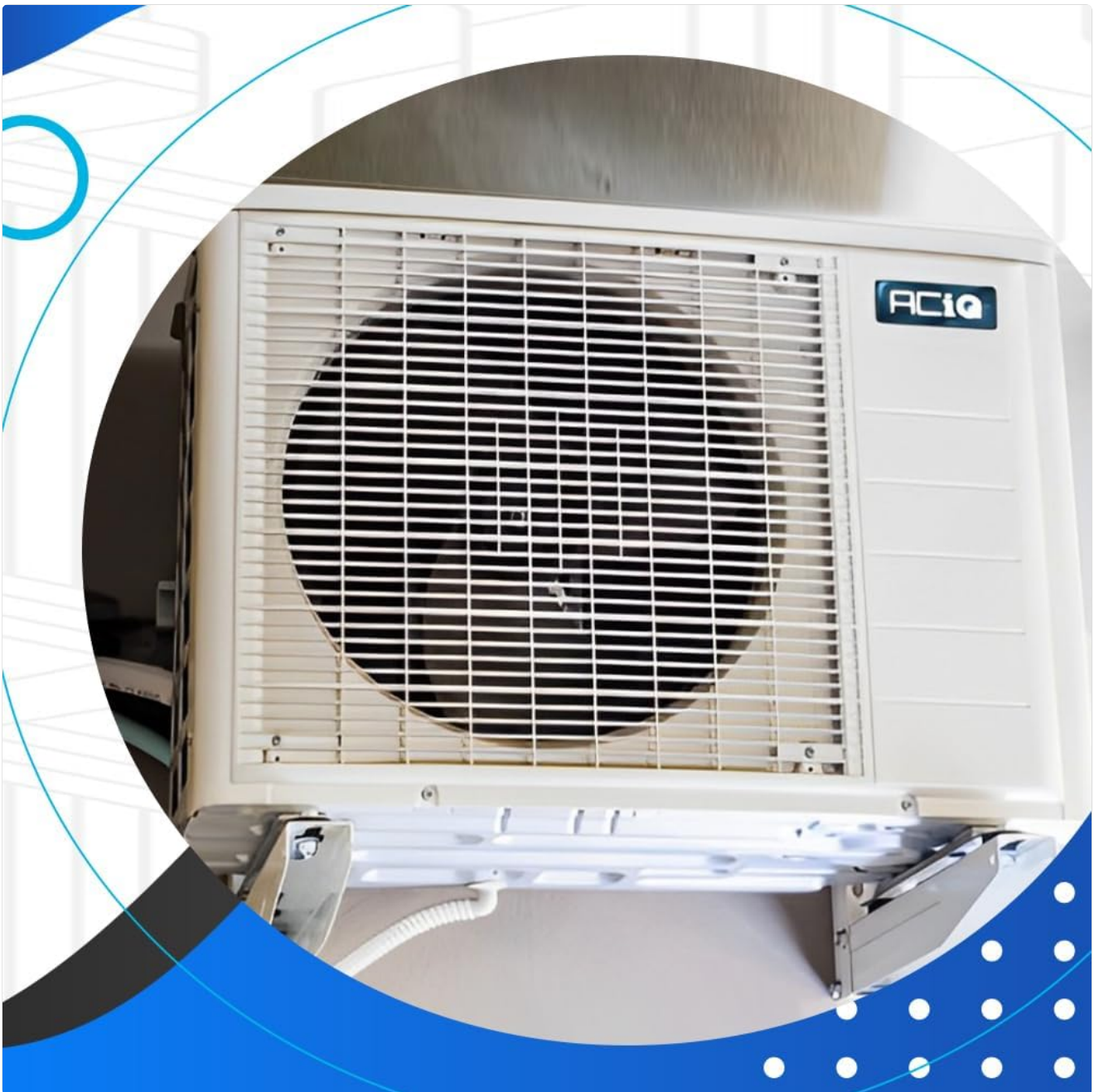
Figure 6.1: A close-up view of the ACiQ outdoor unit, highlighting the fan and condenser coil, which require periodic cleaning for optimal performance.
