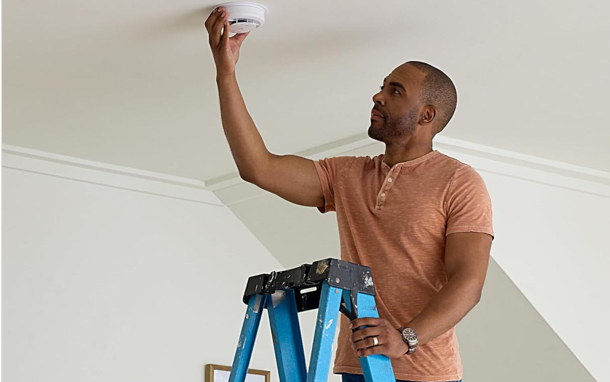
**Image Description:** A man standing on a blue step ladder, reaching up to install a white Kidde 30CUDR smoke and carbon monoxide detector onto a white ceiling. The image illustrates the simple twist-and-click installation process.
