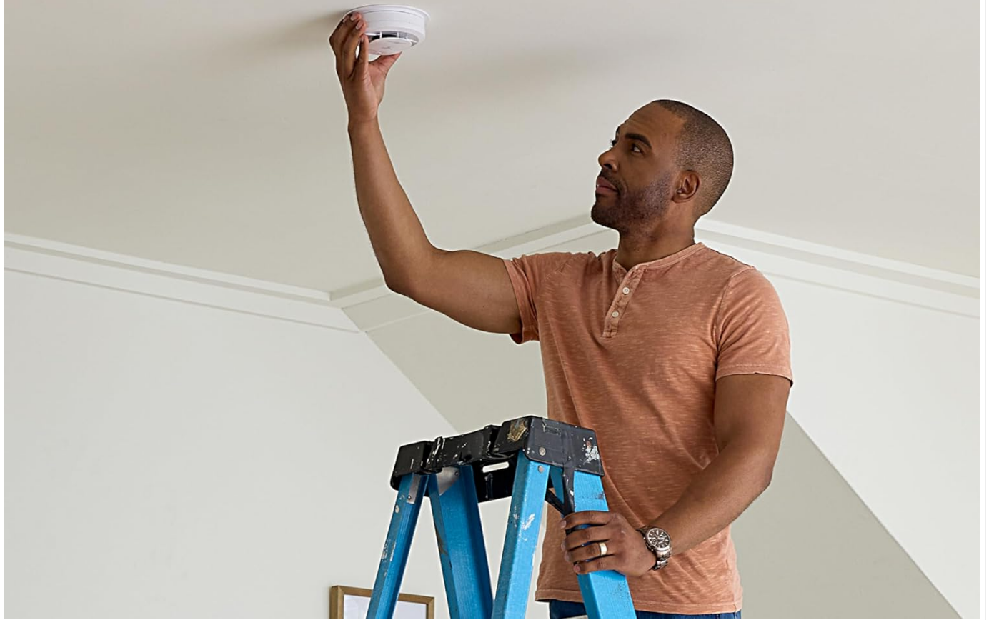
Image 4: Simple installation process showing a person attaching the detector to the ceiling using the twist-and-click mounting bracket.
