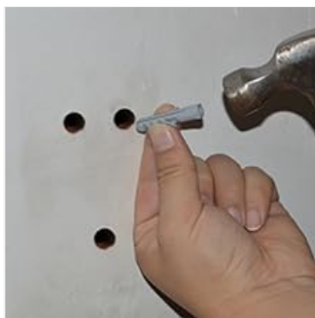
Figure 5.7: Hoist hole installation method.
