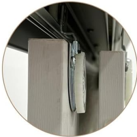
Image 5.1: Key hardware components include quiet-operating rollers, stability-enhancing floor guides, and robust tracks.
