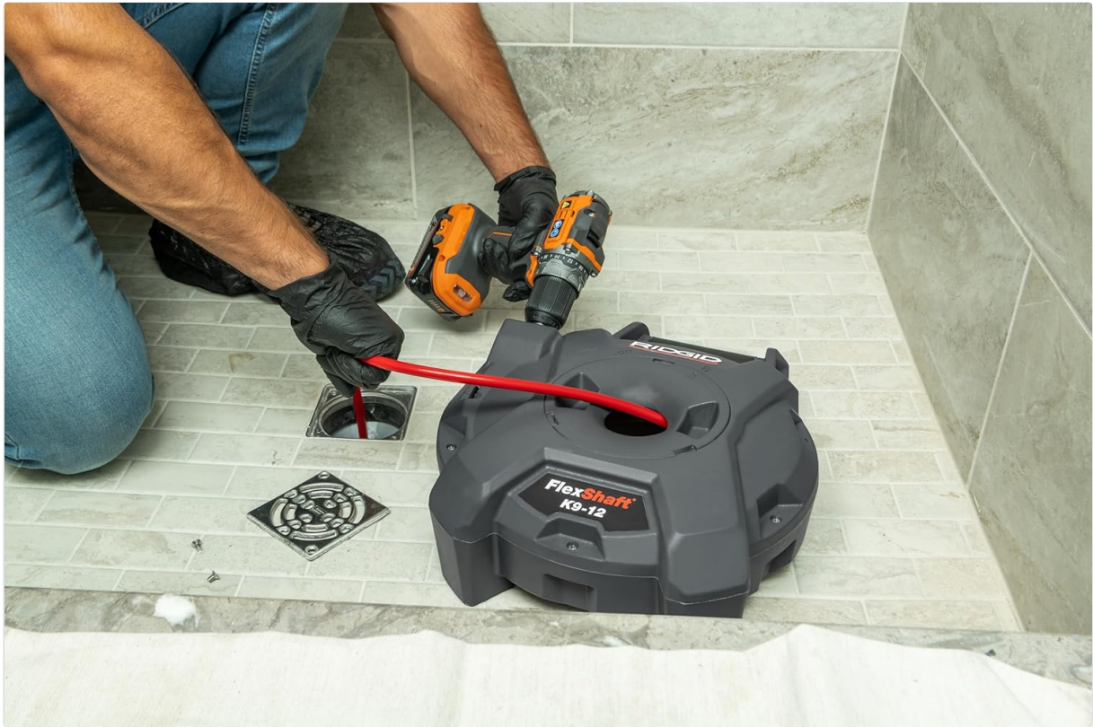
Figure 3.1: A user connecting a cordless drill to the FlexShaft K9-12 machine, positioned next to a shower drain for cleaning.
