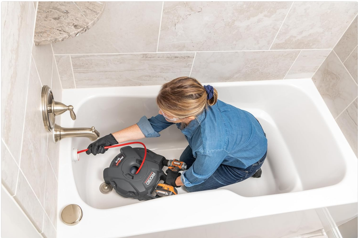
Figure 4.2: A user operating the FlexShaft K9-12 machine to clear a blockage in a bathtub drain.
