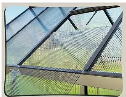
Figure 3: Detail of polycarbonate panels inserted into the frame.
