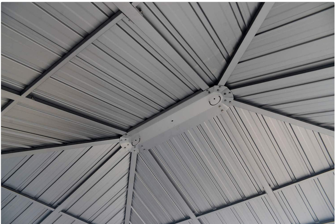
Image: Underside view of the galvanized steel roof, showing the internal support structure and panel connections.
