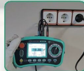
Loop test from a wall socket
