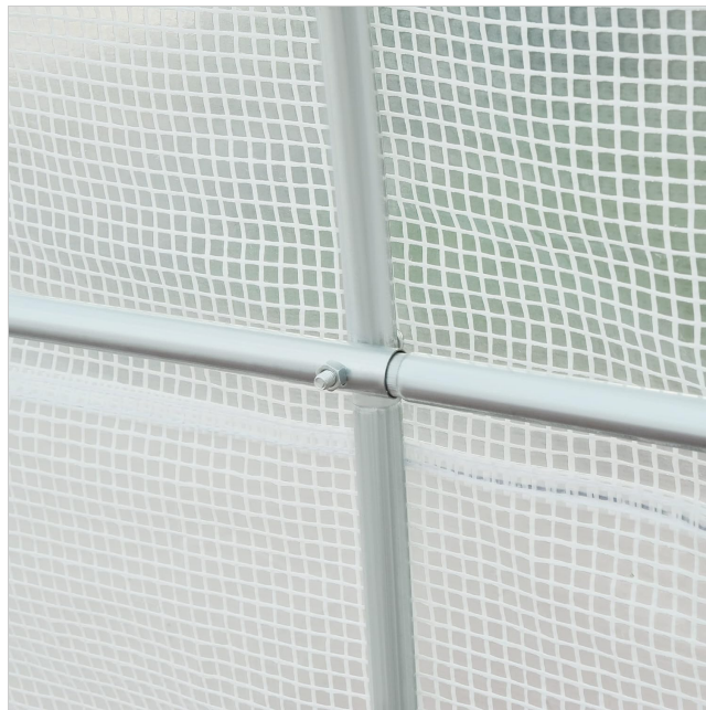
Image: Detail of a steel frame joint.
