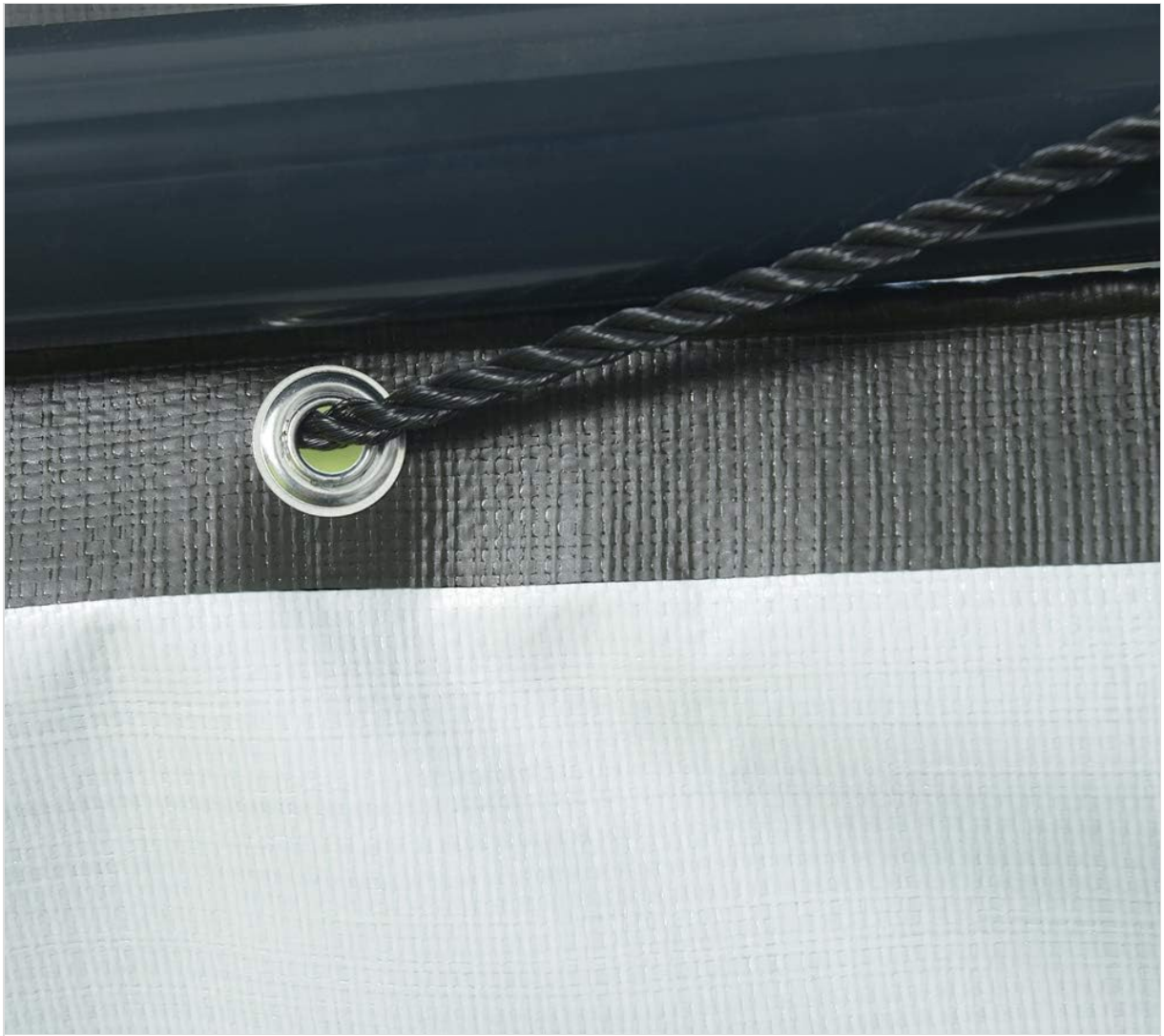
Image 3: Detailed view of the lacing rope used to secure the enclosure panels to the corral frame.
