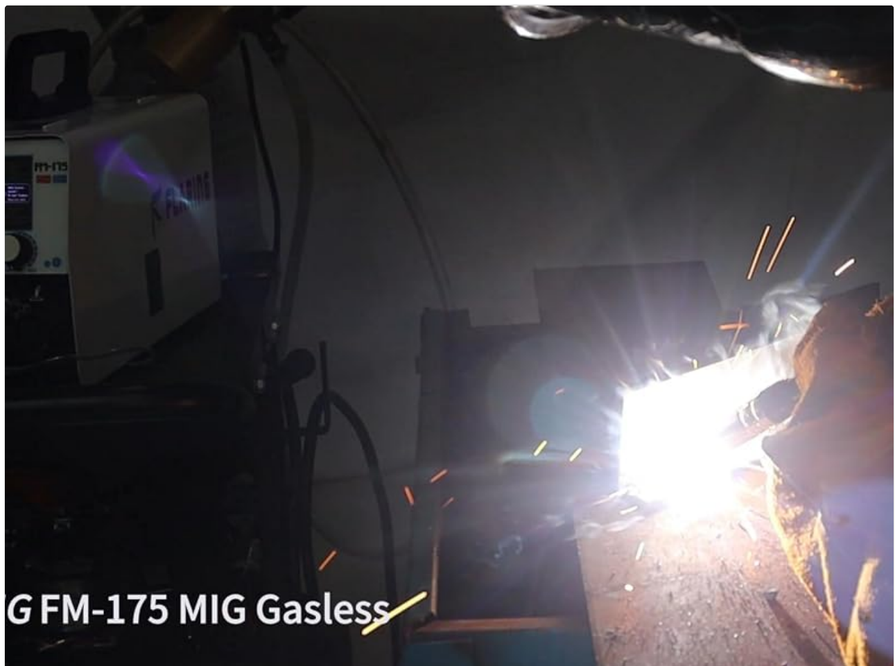
Figure 5.4: Demonstrating MIG Gasless welding with the FLARING FM-175.
