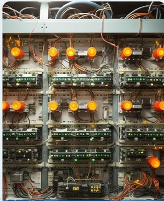
Electric power metering system
