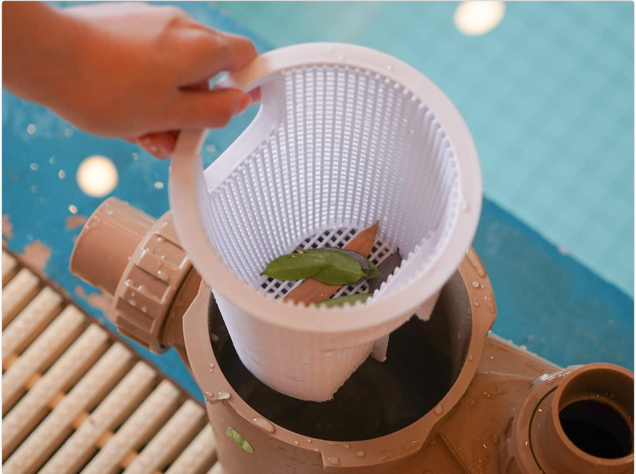
Image 6.1: Cleaning Strainer Basket. A hand lifting the white strainer basket, containing leaves and debris, from the pump's housing, illustrating the ease of maintenance.
