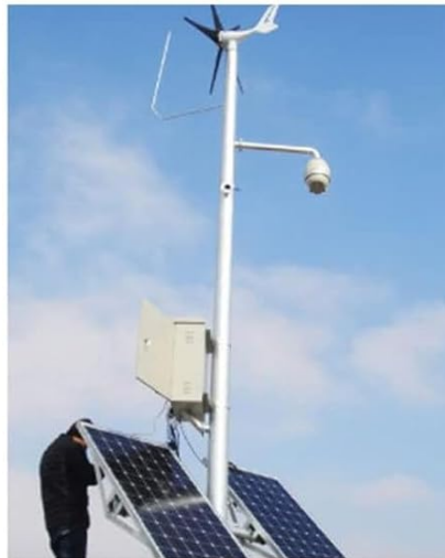
Wind solar hybrid monitoring system
