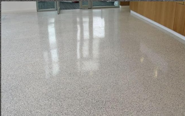
terrazzo floor grinding
