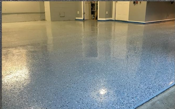
renovation of epoxy floor
