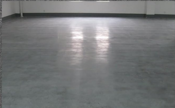
concrete floor grinding
