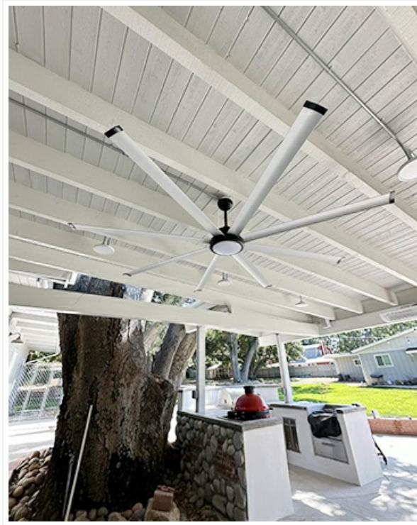
Figure 4.1: Downrod and Sloped Ceiling Mounting Options. Note: Sloped ceiling mount is suitable for angles up to 15 degrees.
