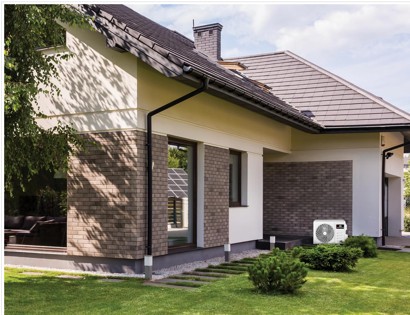
Image 4.2: Example of an outdoor unit placed on the ground next to a residential building.
