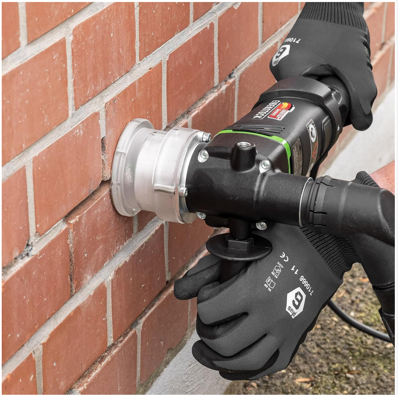
Figure 5: The Eibenstock EFU 1200 being used to mill a joint on a brick wall, demonstrating proper handling with both hands and dust extraction.
