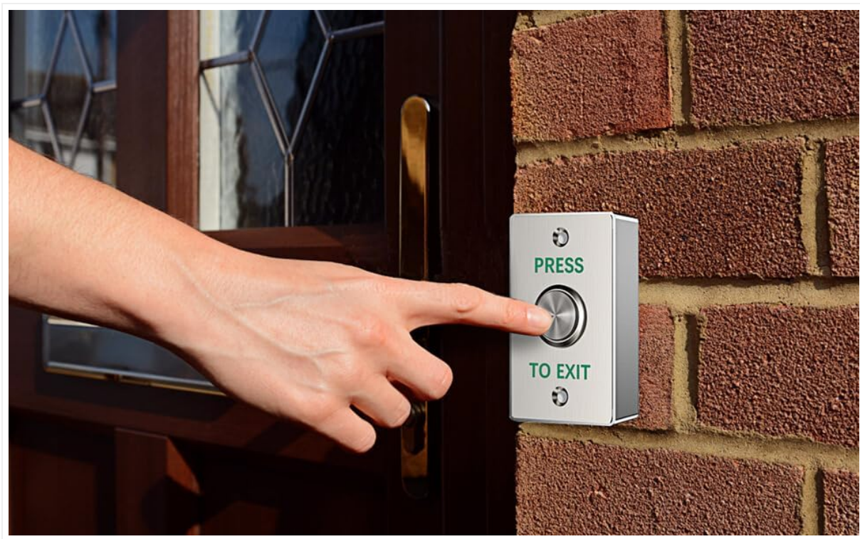
Figure 5: A hand demonstrating the operation of the Push to Exit Button, installed on a brick wall next to a door.
