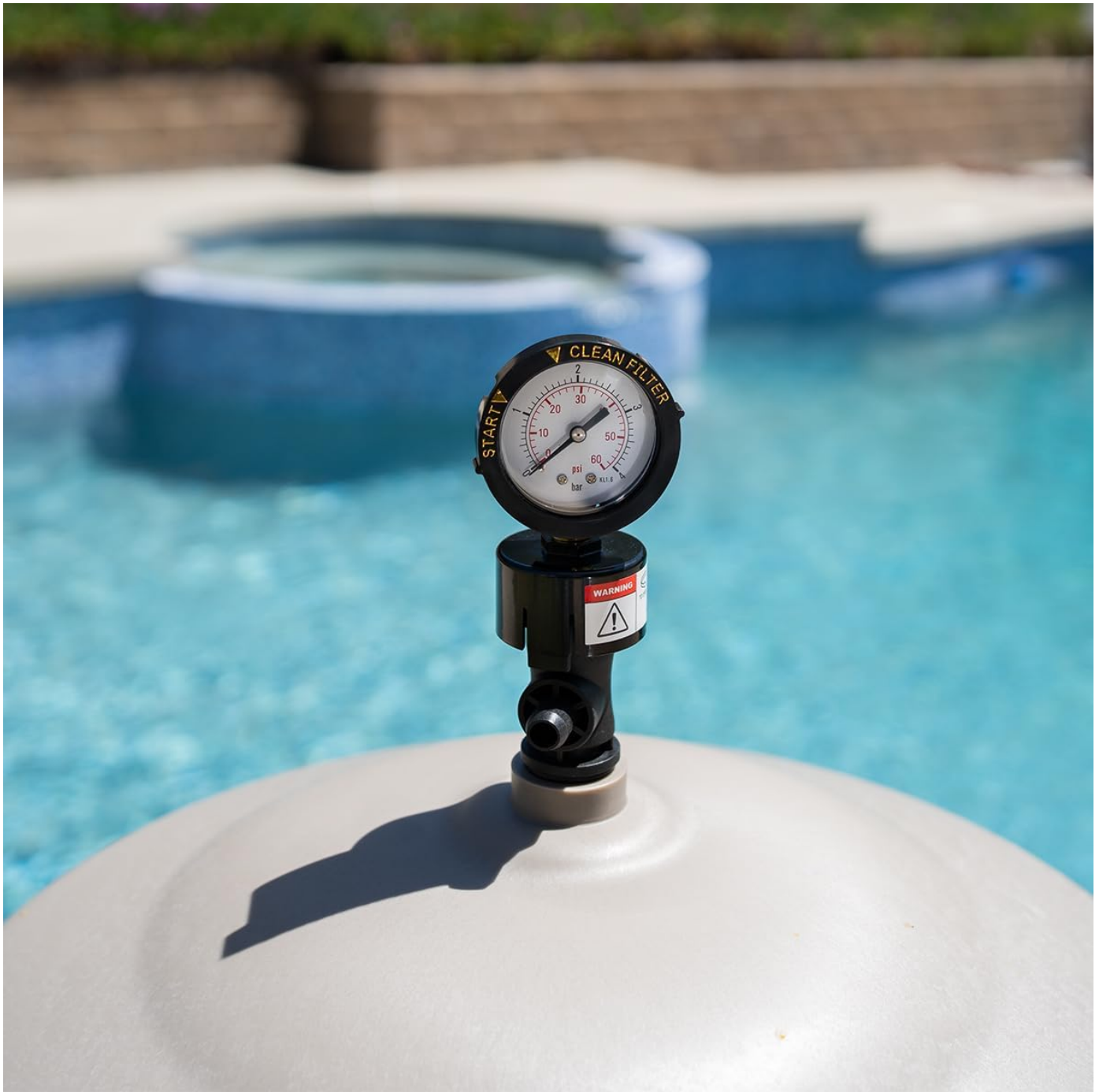
Image 5.1: Pressure gauge indicating filter status.
