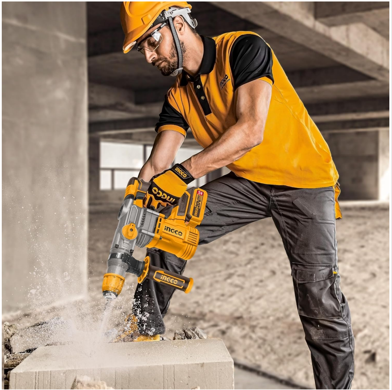
Image 5.2: An operator demonstrating hammer drilling into a concrete surface.
