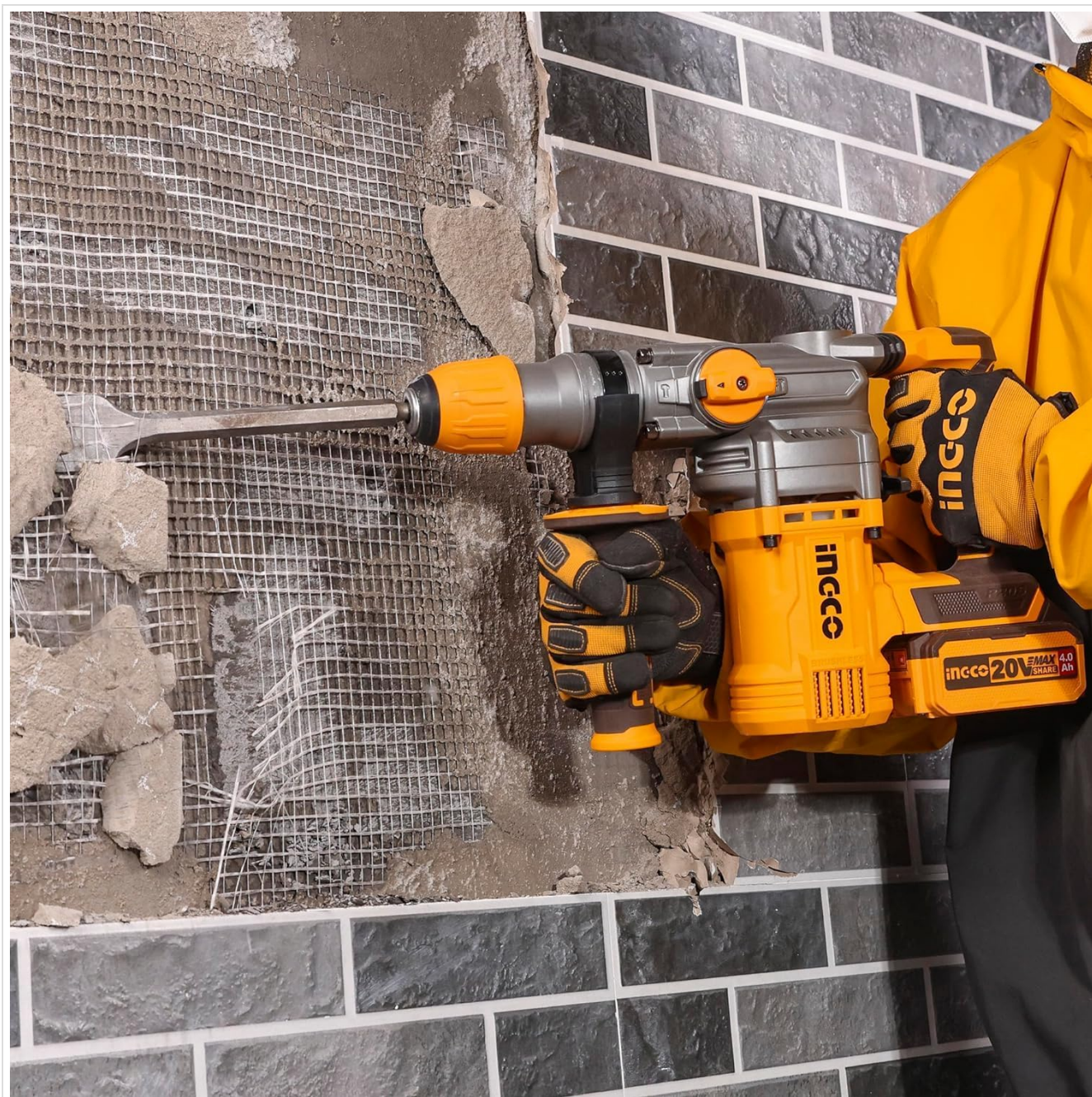
Image 5.4: An operator performing chiseling work on a wall with the rotary hammer.
