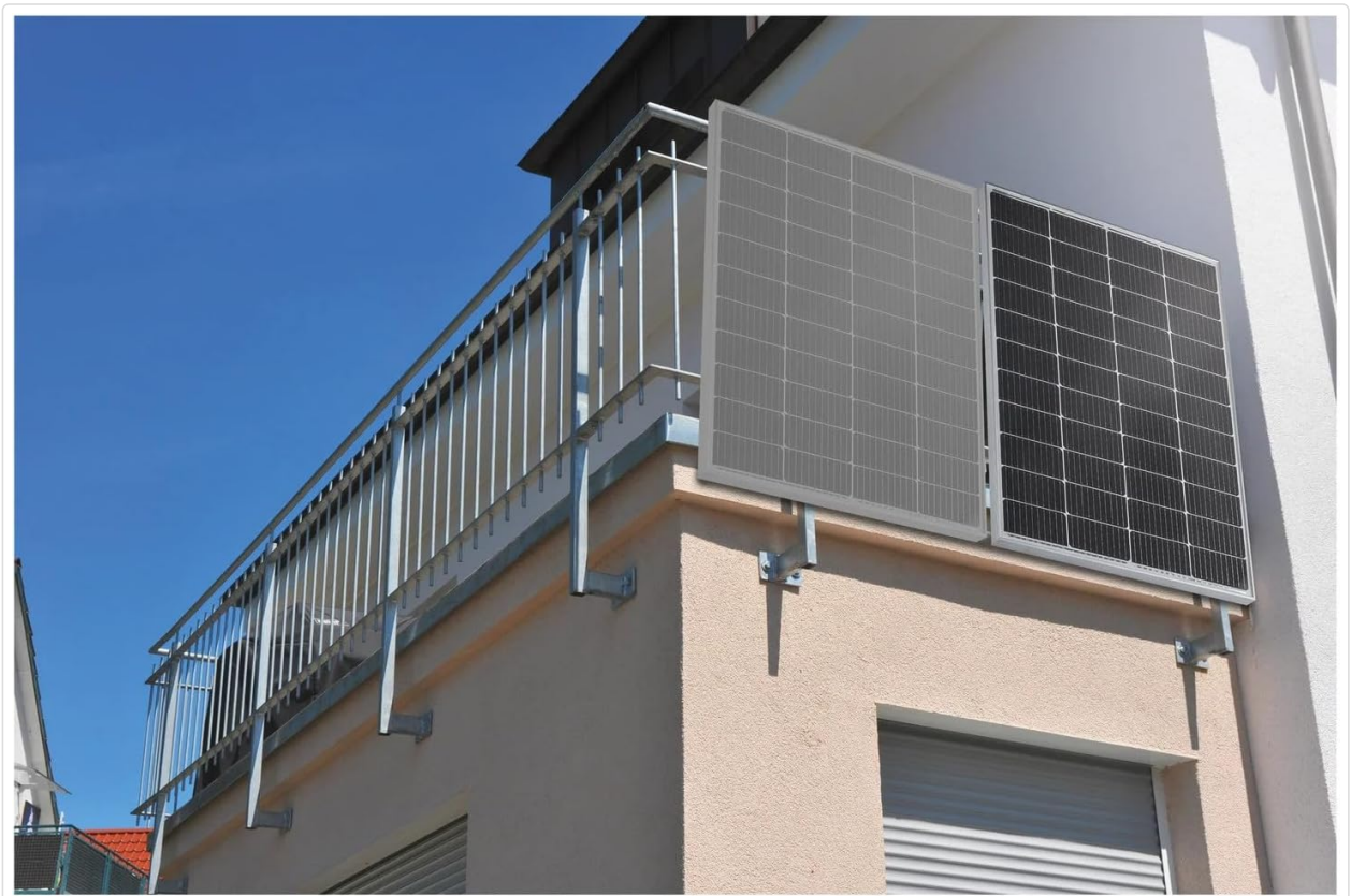
Image: An example of a dual solar panel installation on a balcony.
