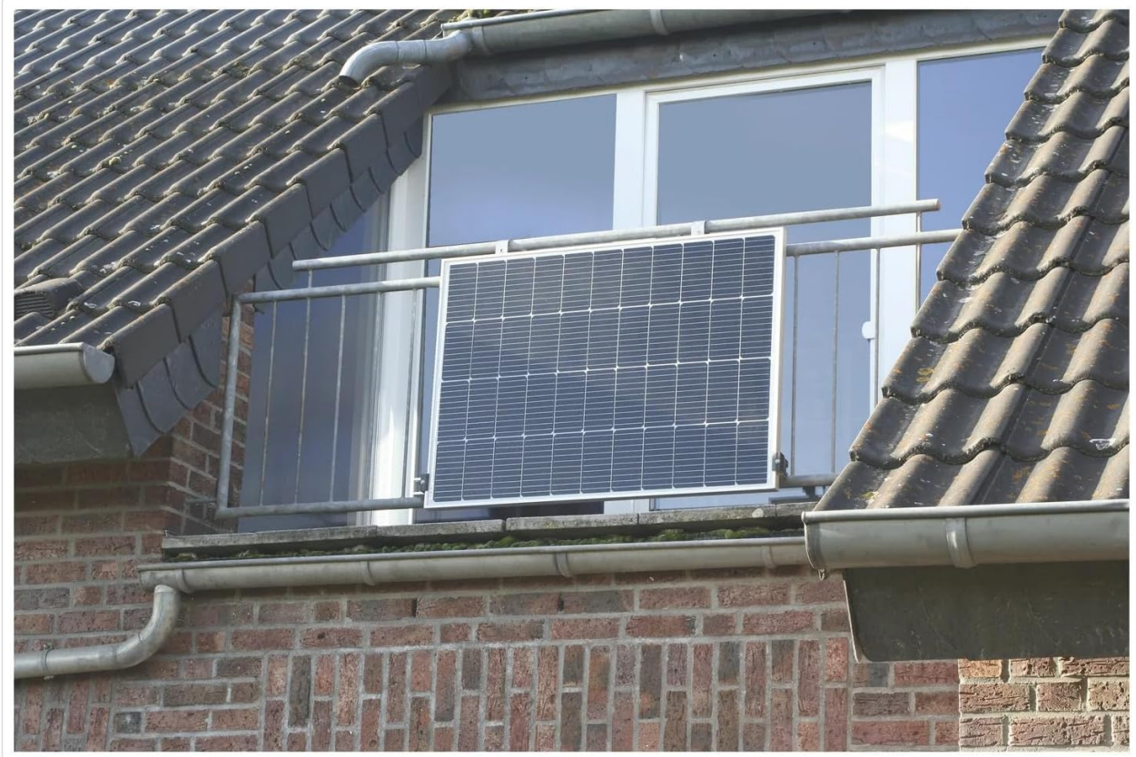
Image: Solar panel installed horizontally on a balcony railing.
