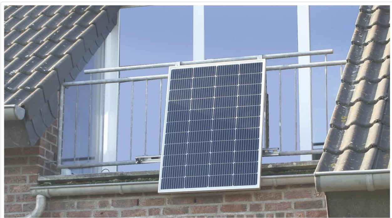
Image: Solar panel installed horizontally on a balcony railing.
