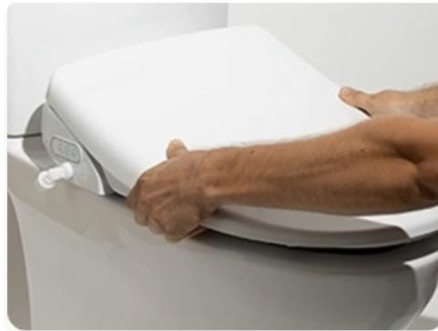
Image: A person's hands unscrewing and lifting an existing toilet seat from the toilet bowl.
