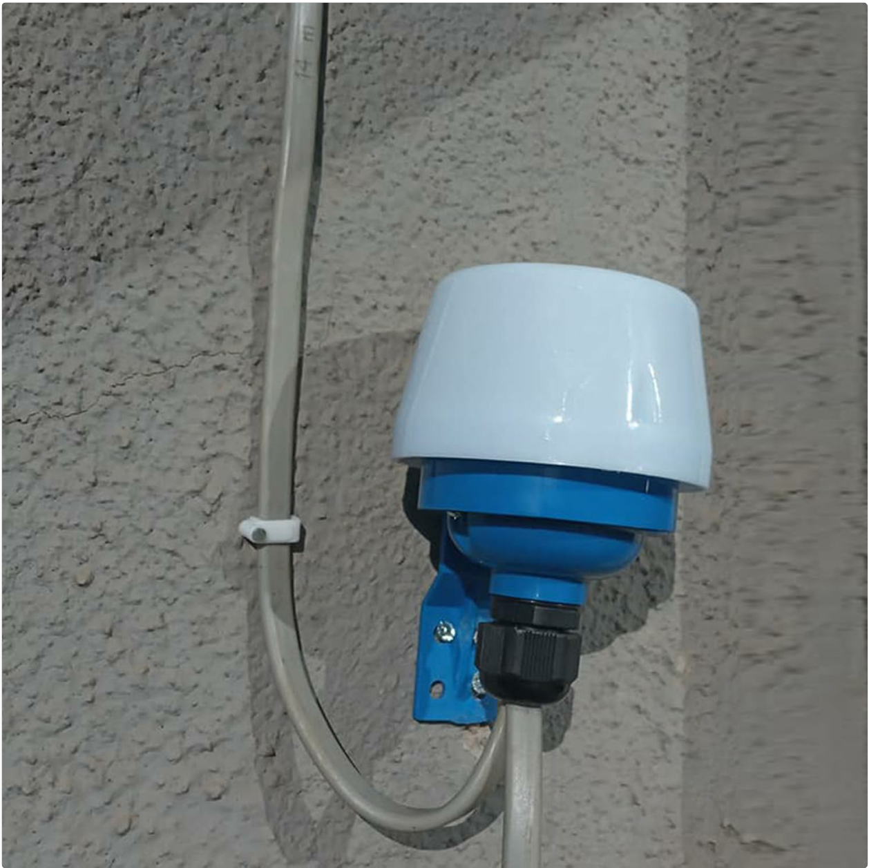
Image 7.3: Example of a correctly installed photocell sensor switch on an exterior wall.
