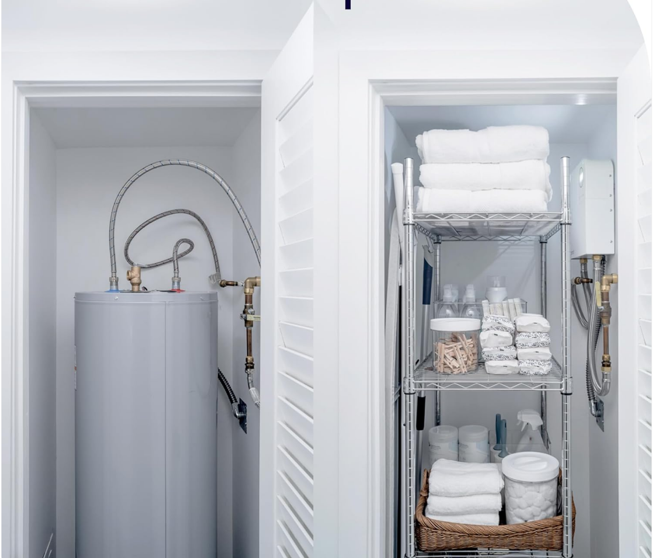
Figure 5: Visual comparison demonstrating the space-saving advantage of the tankless water heater over a traditional tank unit.
