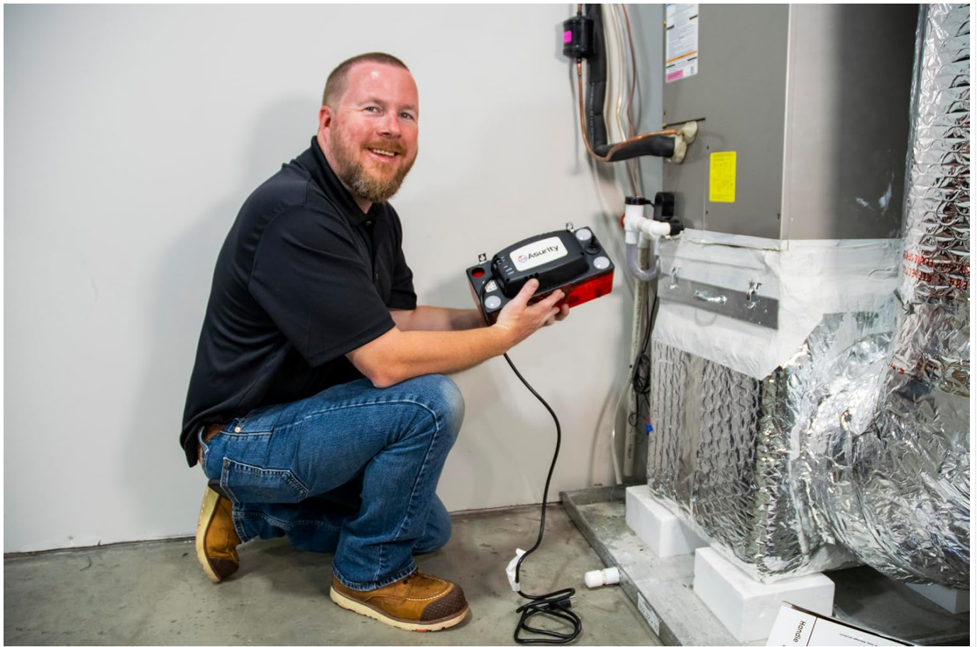
Figure 5: The pump in an operational setup, showing connections.
