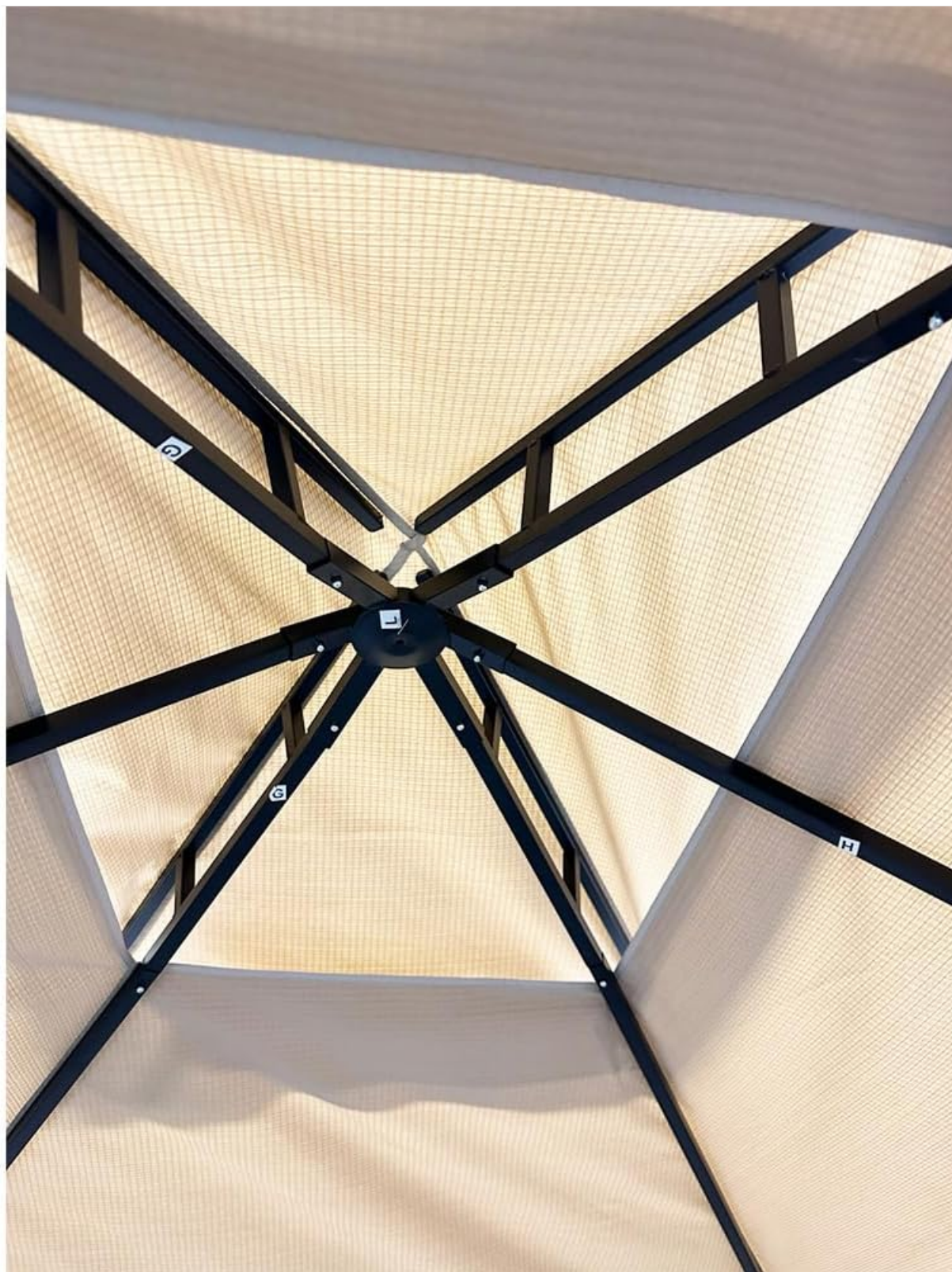
Image 2.2: Detail of the central frame connection point, illustrating how the canopy attaches to the gazebo structure.
