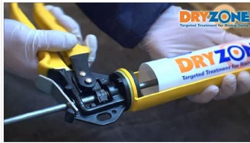
Figure 4: Inserting the nozzle and using a caulk gun for cream injection.
