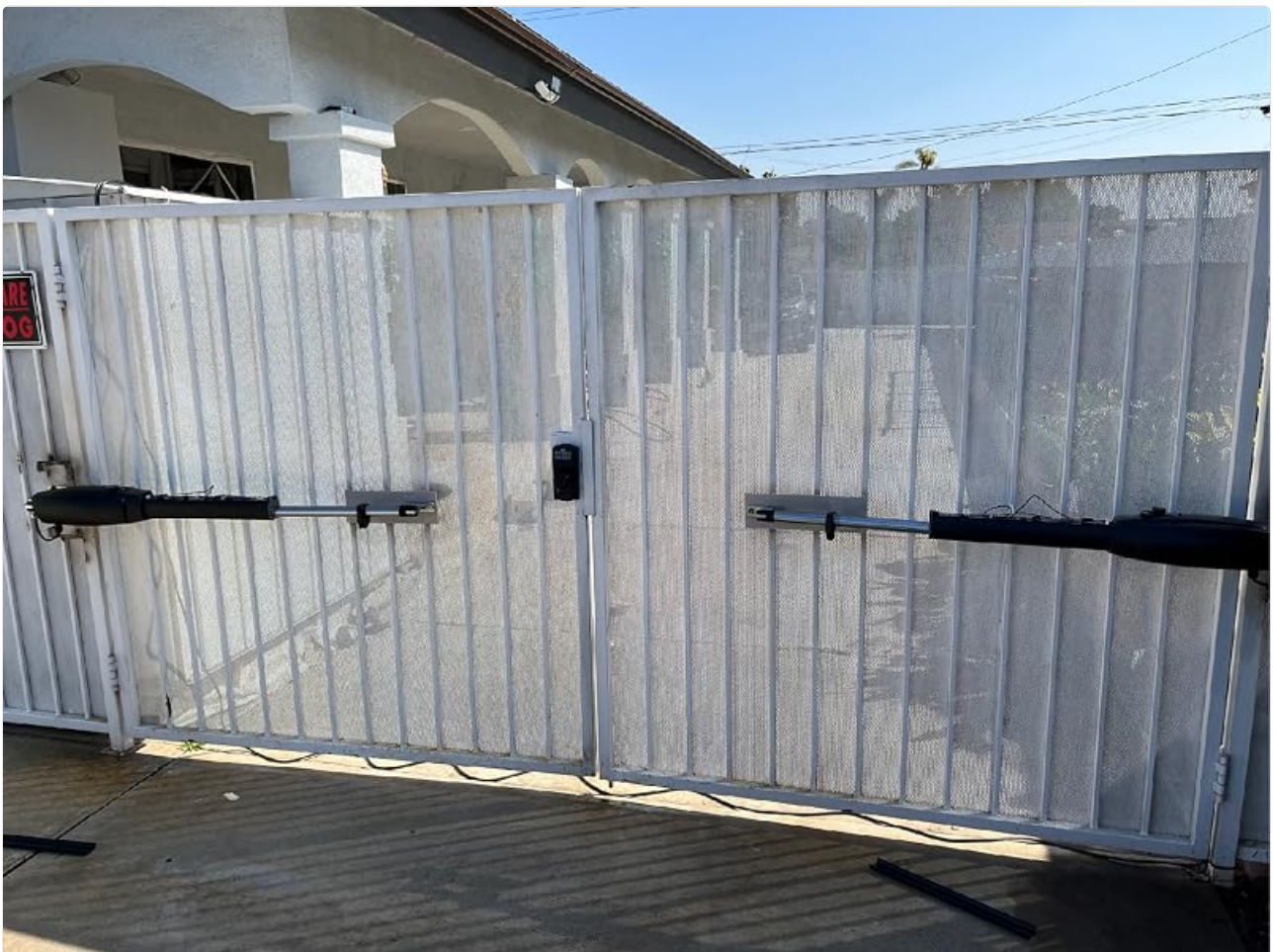
White Metal Gate Installation
