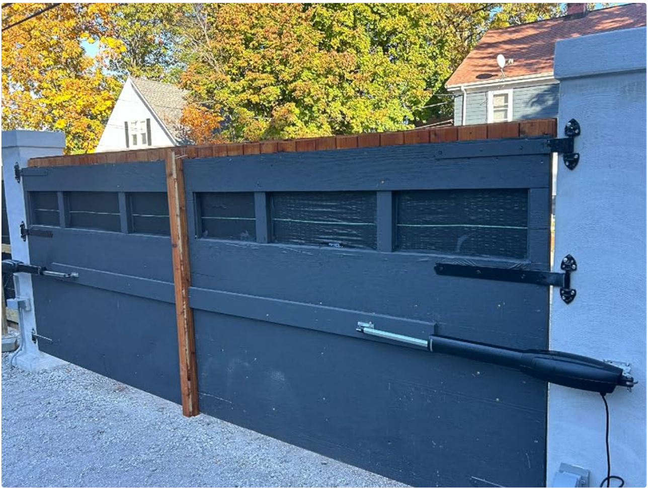
Large Wooden Gate Installation
