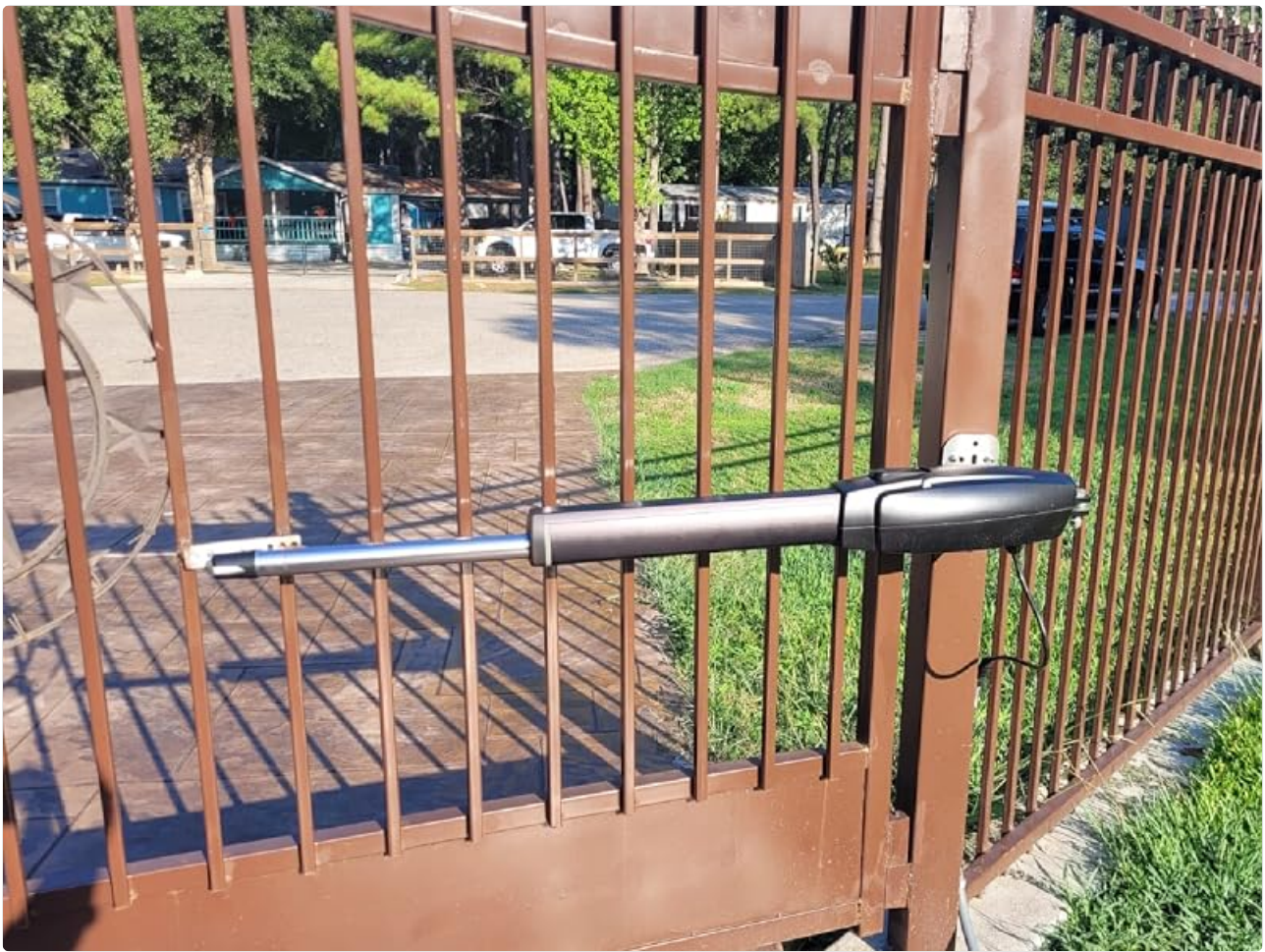
Metal Gate Installation
