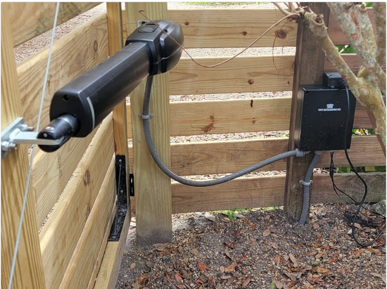
Wooden Fence Gate Installation
