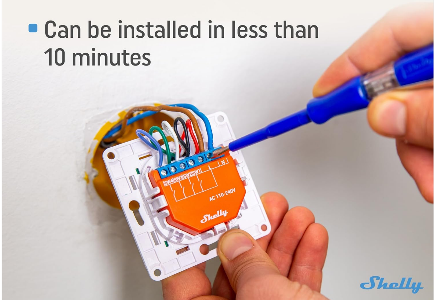
Image 3: Shelly Plus i4 UL being installed behind a wall switch. This image illustrates the compact size of the device, allowing it to fit into a standard electrical box behind a switch.
