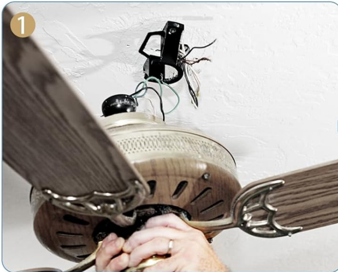
1 Disconnect the ceiling fan wiring
