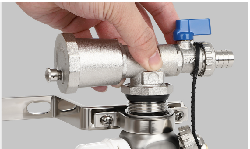
Figure 6: Attaching the automatic air vent and drain valve to the manifold.
