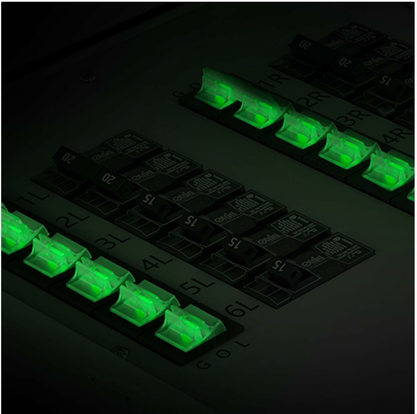
Image: Close-up view of the rocker switches on the transfer switch, showing the green illumination when a circuit is active
