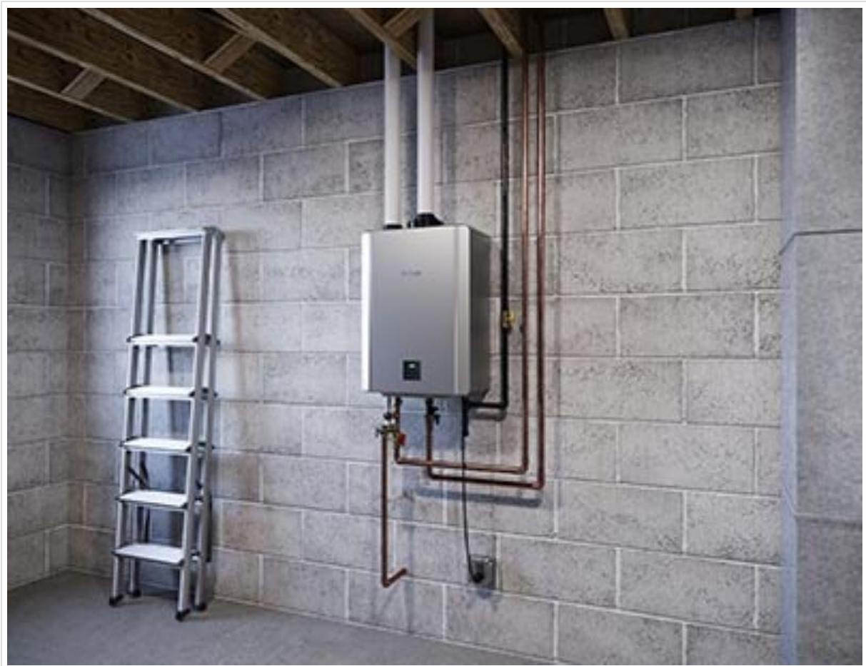
Figure 4.1: Example of an indoor installation, showing the unit mounted on a wall in a utility space.
