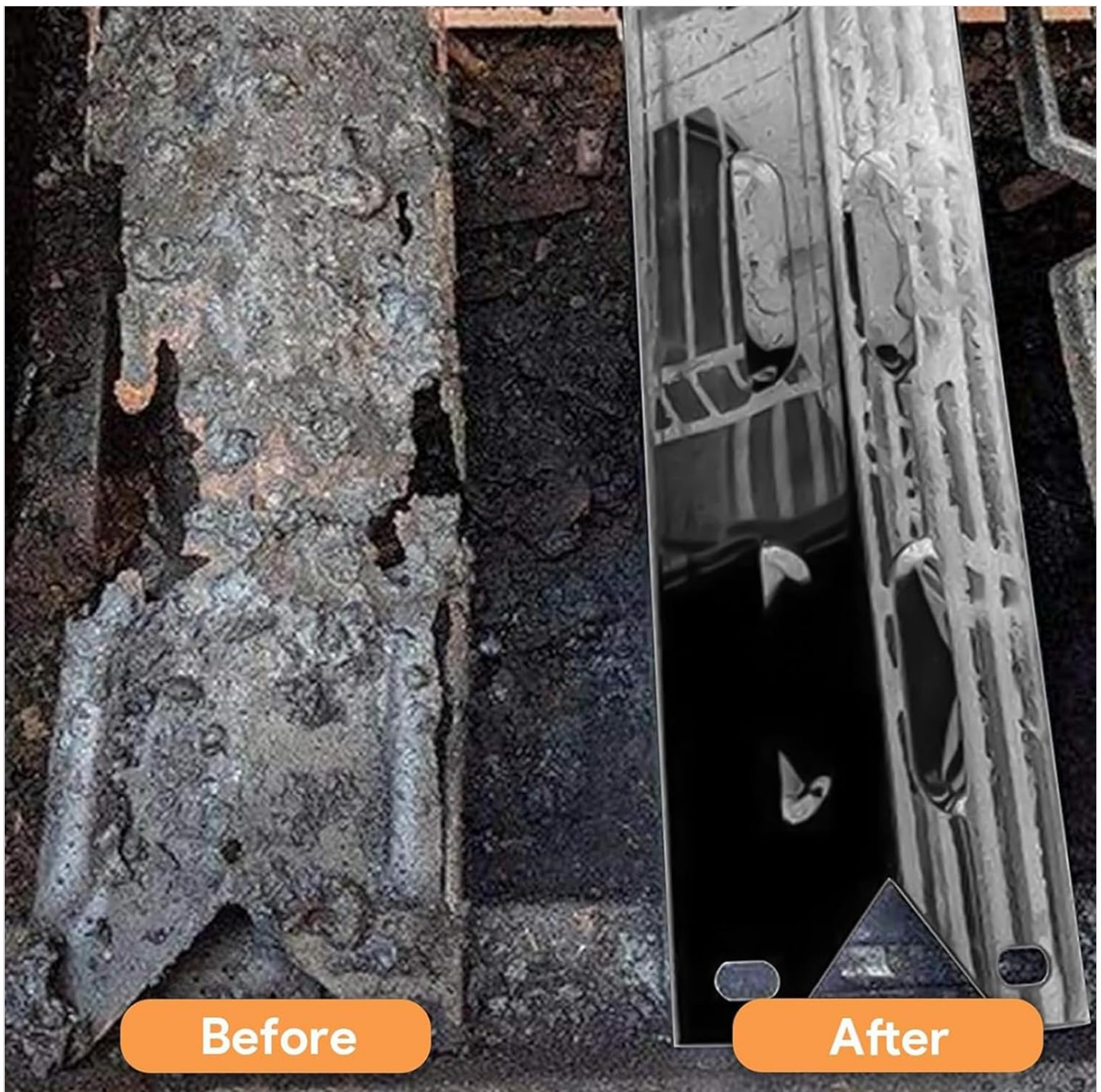
Image: A side-by-side comparison showing a heavily corroded old heat plate next to a new, clean replacement heat plate, highlighting the improvement after replacement.
