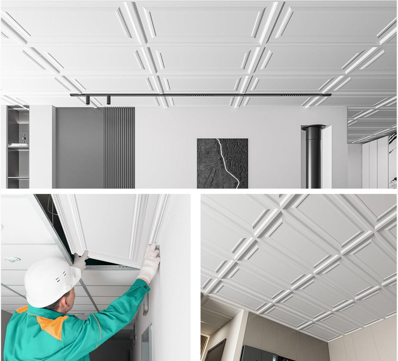
Image 4.2: A worker demonstrating the installation of an Art3d ceiling tile into a T-bar grid, highlighting the simple lay-in process.
