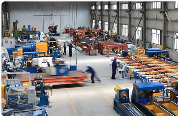
Industrial Plant Retrofit
