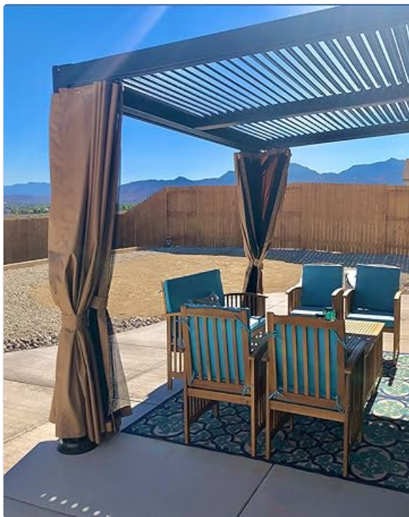
Figure 3.2: Adjustable louvers allowing precise control over sun exposure.
