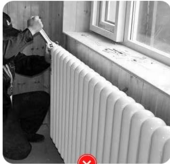
Heating pipe leakage
