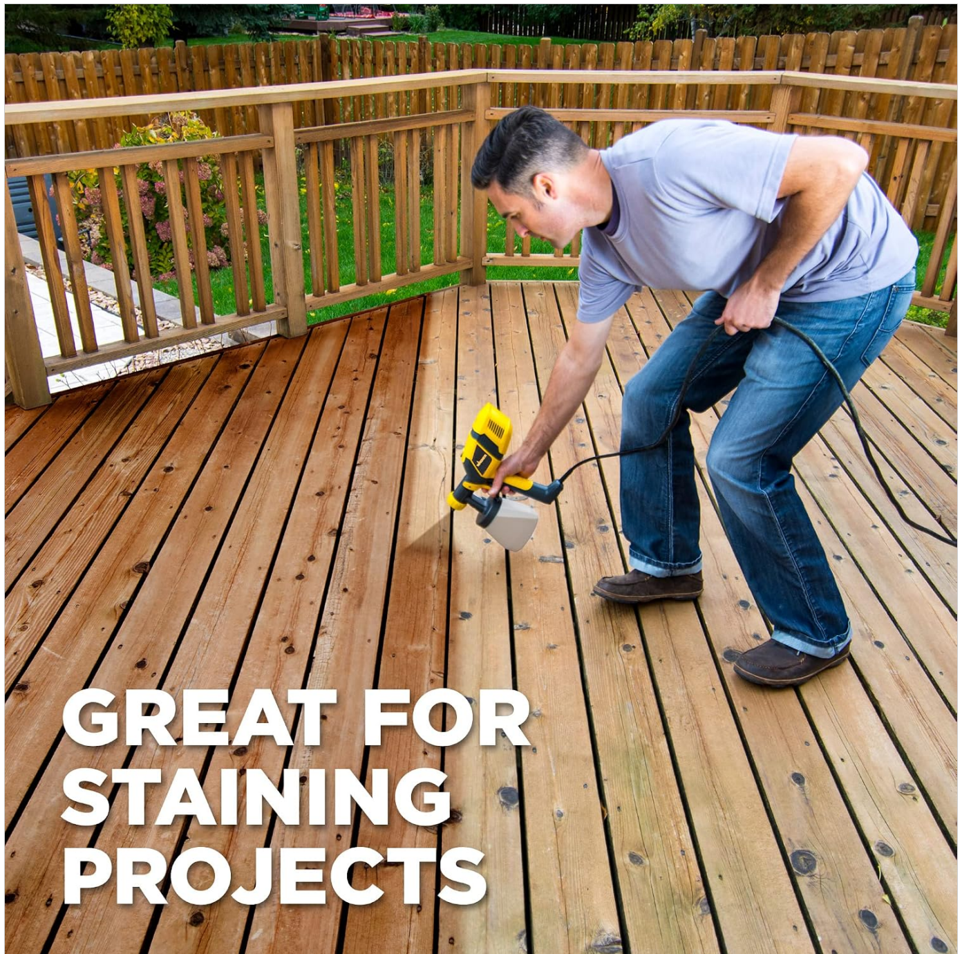
Figure 6: Staining a wooden deck surface
