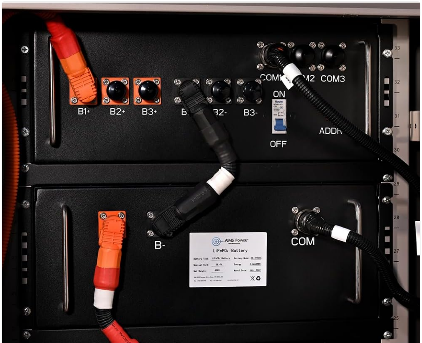
Figure 3: Detailed view of the internal wiring and battery connections. This shows the B+, B-, and COM ports, along with an ON/OFF switch and address settings, indicating the modular nature of the battery system.
