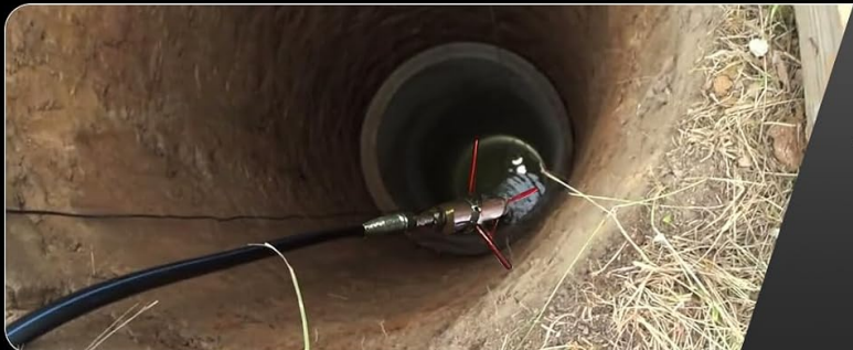
Image 4.6: Demonstrations of the 50ft semi-rigid cable being used with a drain snake, a plastic baseball for centering, and a fish tape for extended reach.
