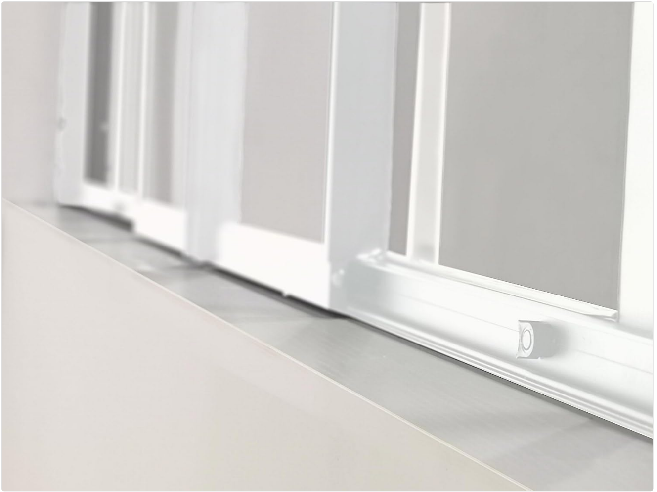
Image: Detailed view of the bottom rail, showing the track for the sliding panels.
