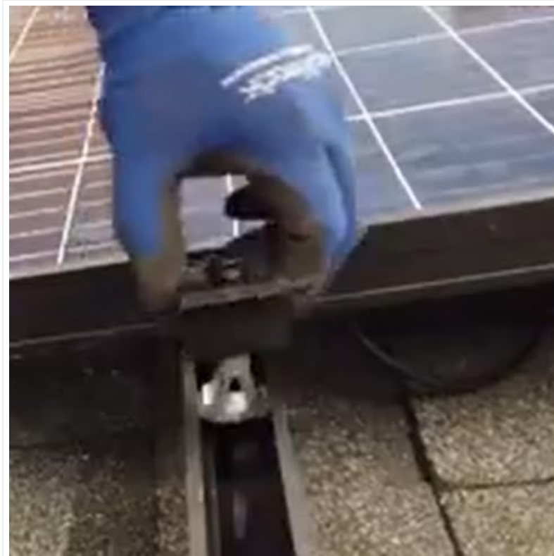
Figure 3: An installer's hand positioning the SnapNrack Ultra Rail Mid Clamp onto the rail system, ready to secure solar panels.
