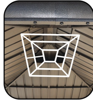
Spoke support beam Tower structure
