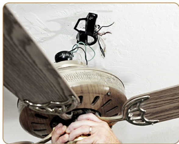
Image: Step 1 - Turn off power to the fan at the circuit breaker.
