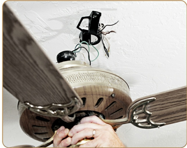
Figure 5: Disconnecting existing ceiling fan wiring.
