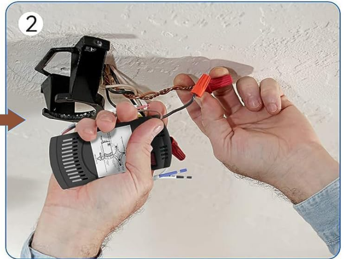
2 Install the controller according to the cable
