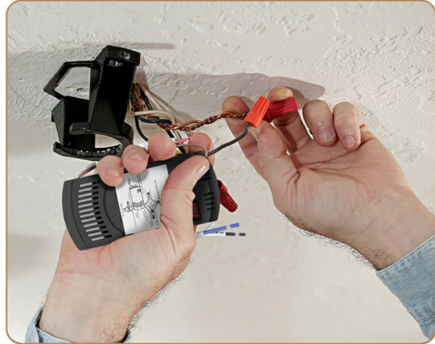
Figure 6: Connecting the receiver to the fan wiring.
