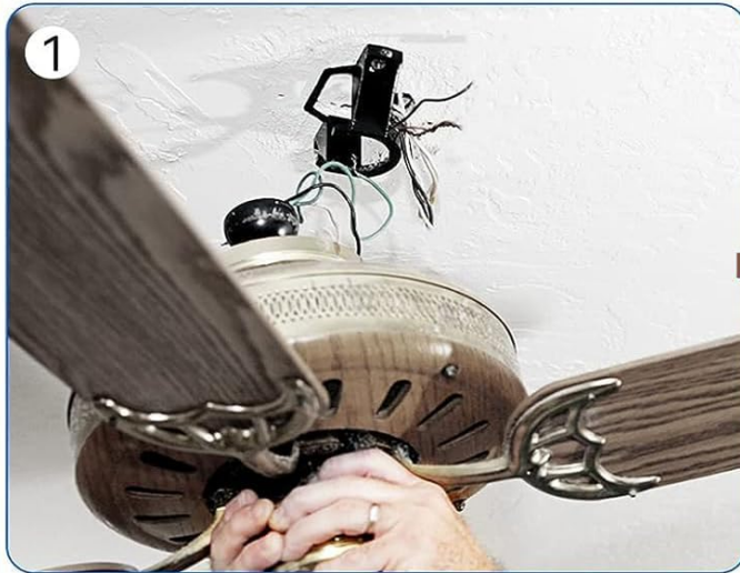
1 Disconnect the ceiling fan wiring
